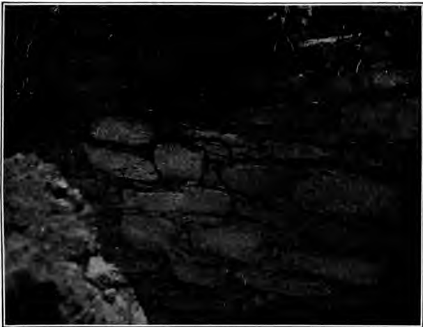
FIG. 21. Construction of wall, ruin at Blue post-office, Blue river.
