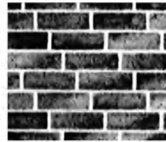
raking stretcher bond
